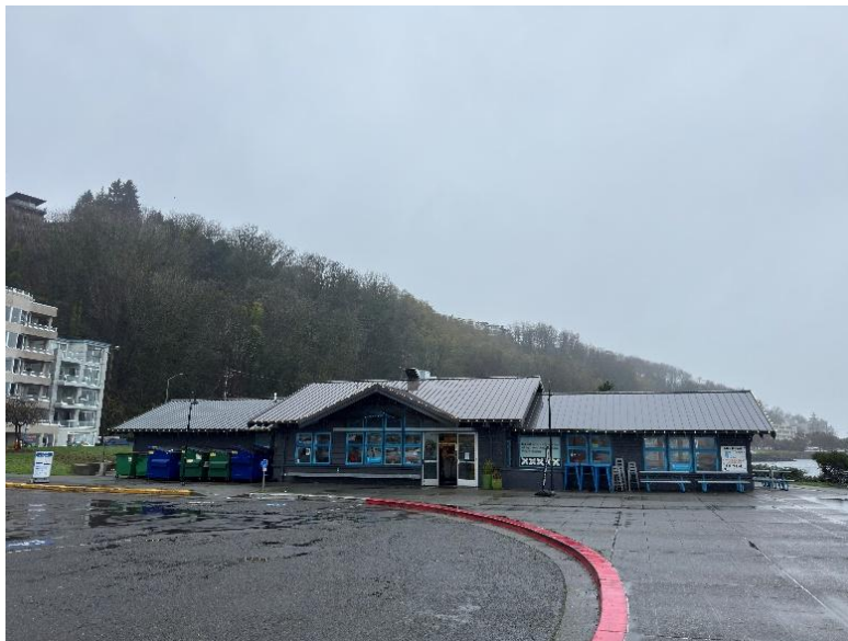
Figure 1 - Exterior Looking North
